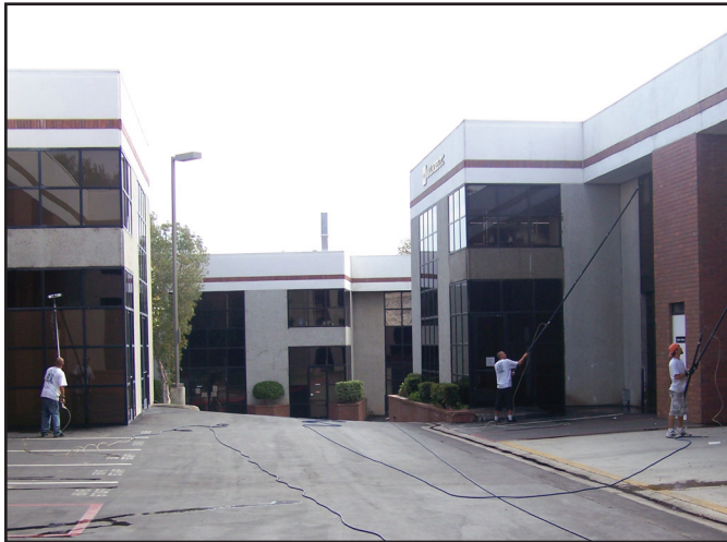
Up to five CarbonTec poles can connect to the pure water tank, allowing several workers to clean at once.
